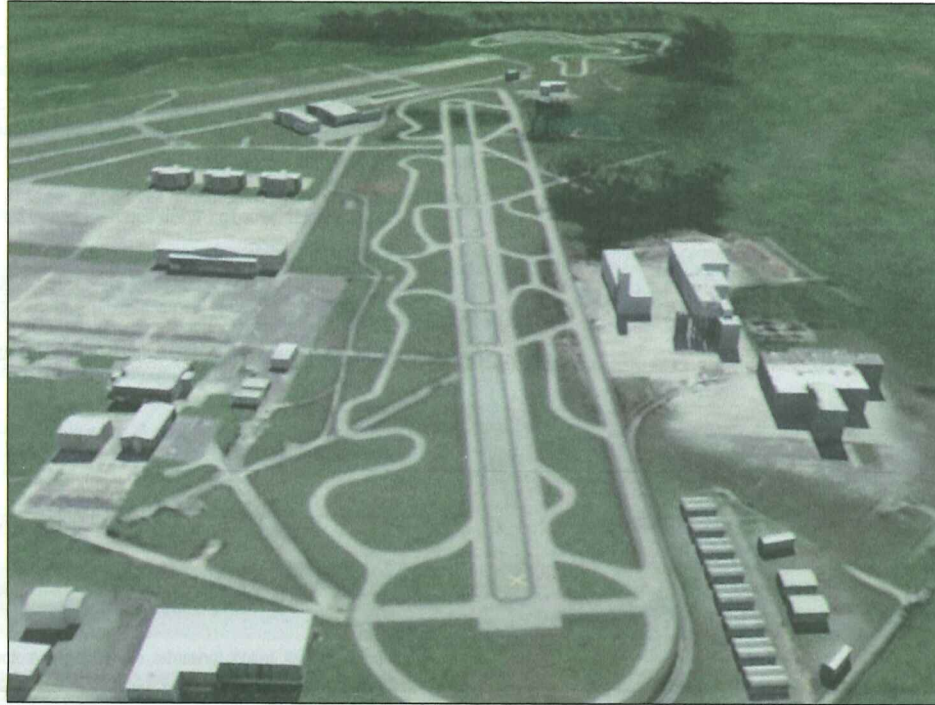
A 5,000-foot runway at SCTAC will be used to test vehicle technology through a new partnership with the Clemson University International Center for Automotive Research. (Image/Provided)
